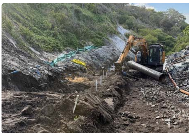
Works to stabilise the bottom of the northern embankment
