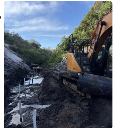
Piling rig on site following rain in June
