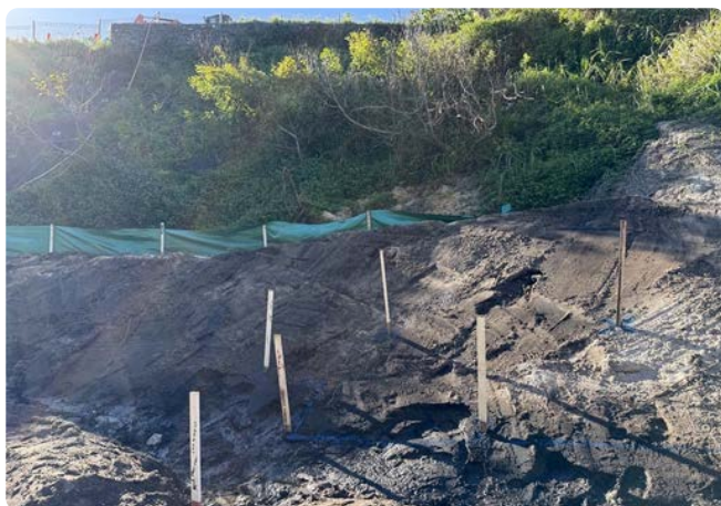
Downslope set out for achors and piling
