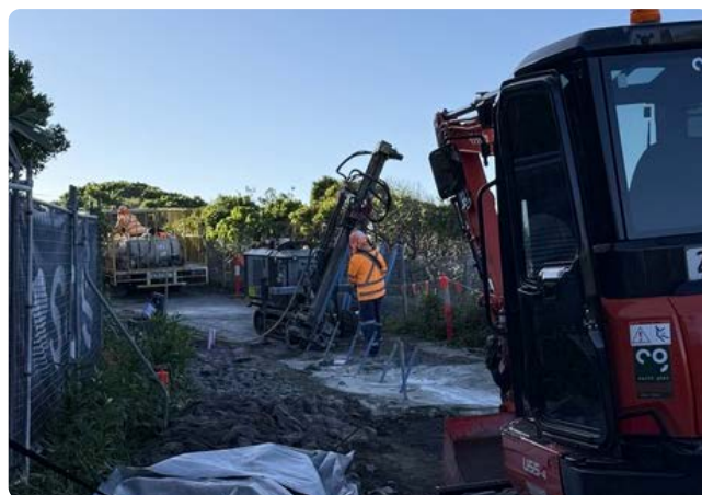
Stabilising anchor micro piles and concrete structure at footpath level
