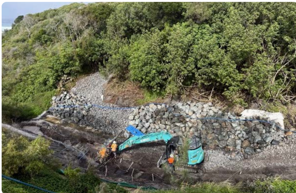
Rock armour on the southern embankment
