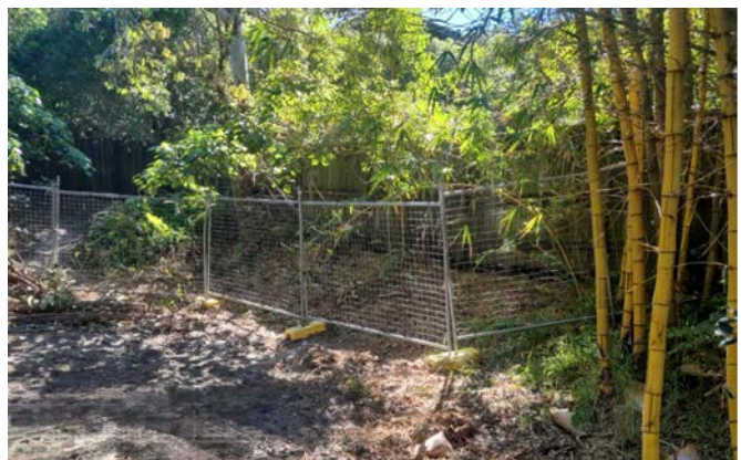
New site fencing
