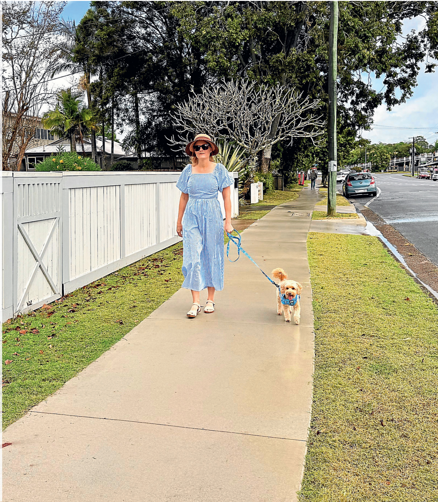
Council has completed a number of pathway upgrades, including Diamond St in Cooroy, as part of its Pathways Renewals Program.
