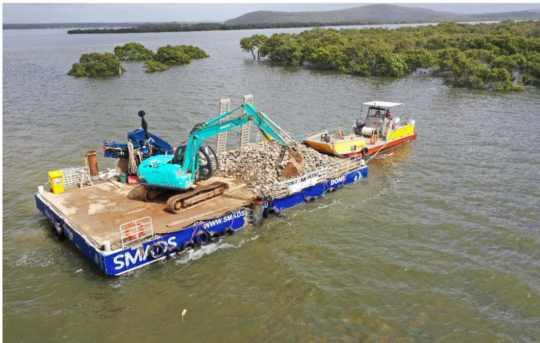
Figure 2: Barge and push vessel used for transporting and deploying substrate on the restoration sites
