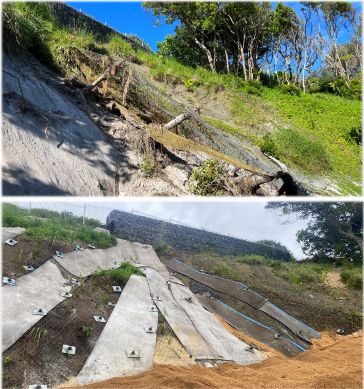
Ross Cres, Slope stabilisation before and emergent works
