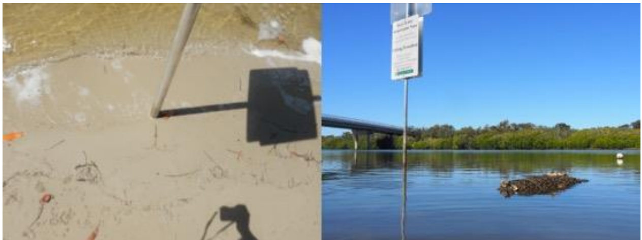
Figure 4 The resulting very small footprint of sign posts following installation by the water jet (left) and a completed oyster reef in Weyba Creek (right).
