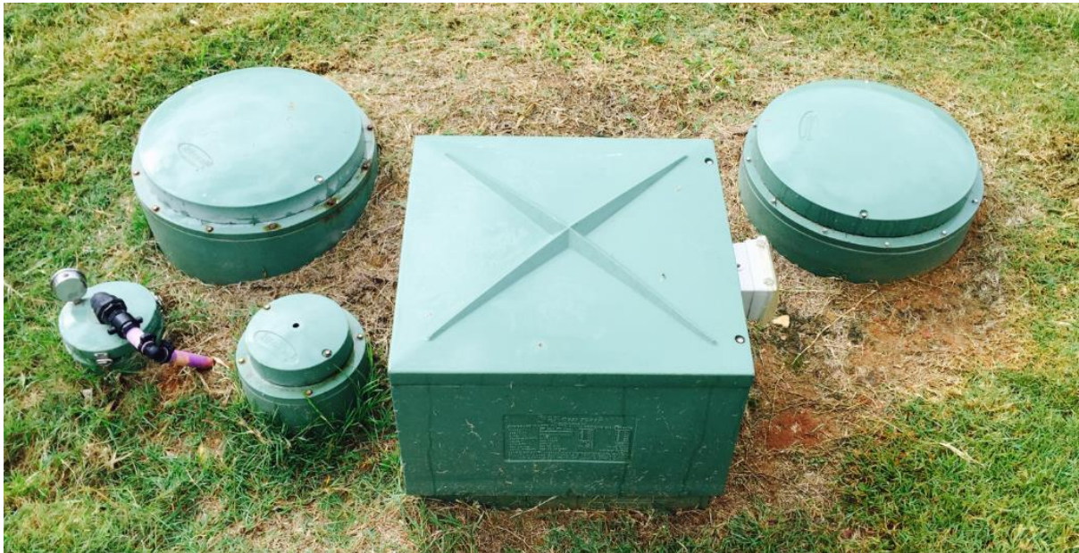
Figure 4 - Aerated treatment plant
