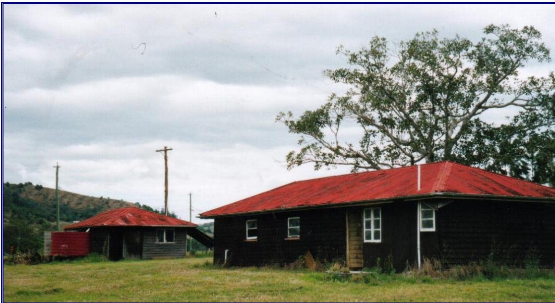
Former farm and dairy buildings on "Mary Waters", corner Bruce Highway and Skyring Creek Road
