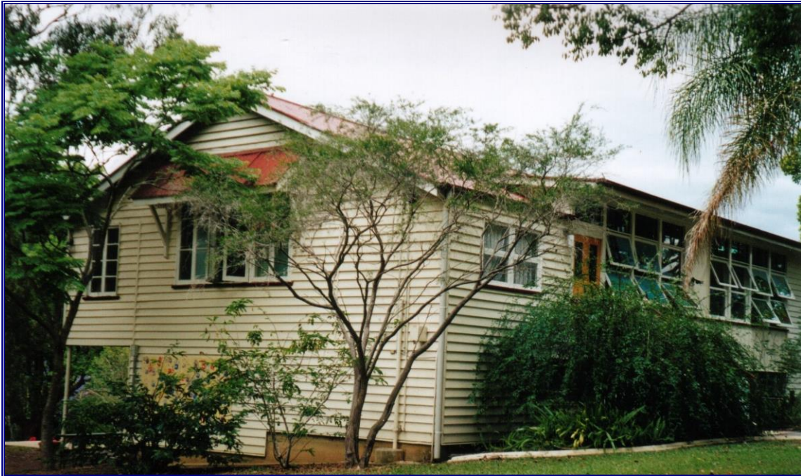
To the left is the Original Federal State Schoolhouse, which is now incorporated into later buildings.
