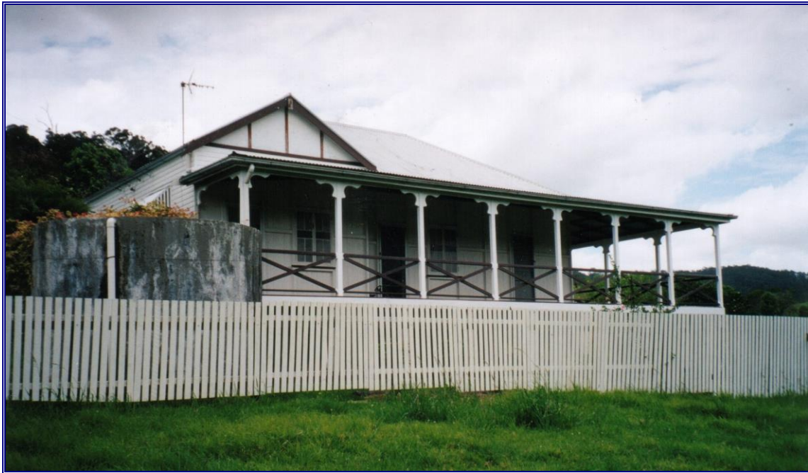
Former Gallen (now McGregor) homestead, Middle Creek Road
