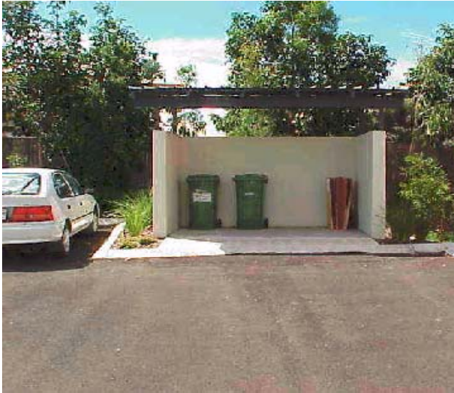
Figure 7.2 An unroofed waste storage area containing a 1100 litre low noise bulk bin suitable for the resort situation. The bin enclosure has a bunded area for bin washing.
