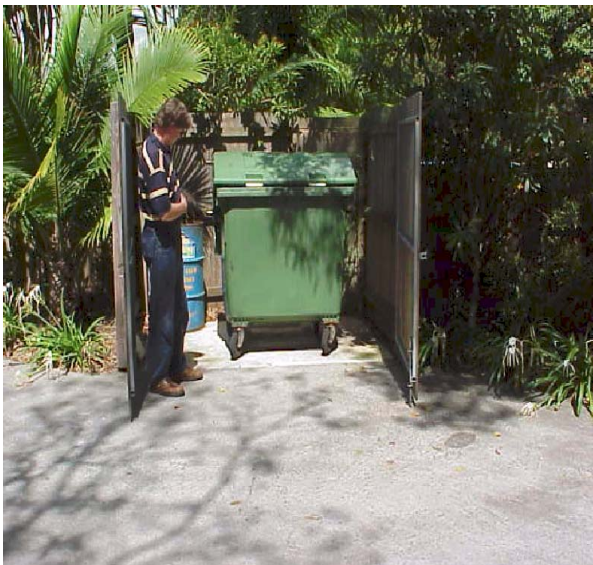
Figure 7.2 An unroofed waste storage area containing a 1100 litre low noise bulk bin suitable for the resort situation. The bin enclosure has a bunded area for bin washing.
